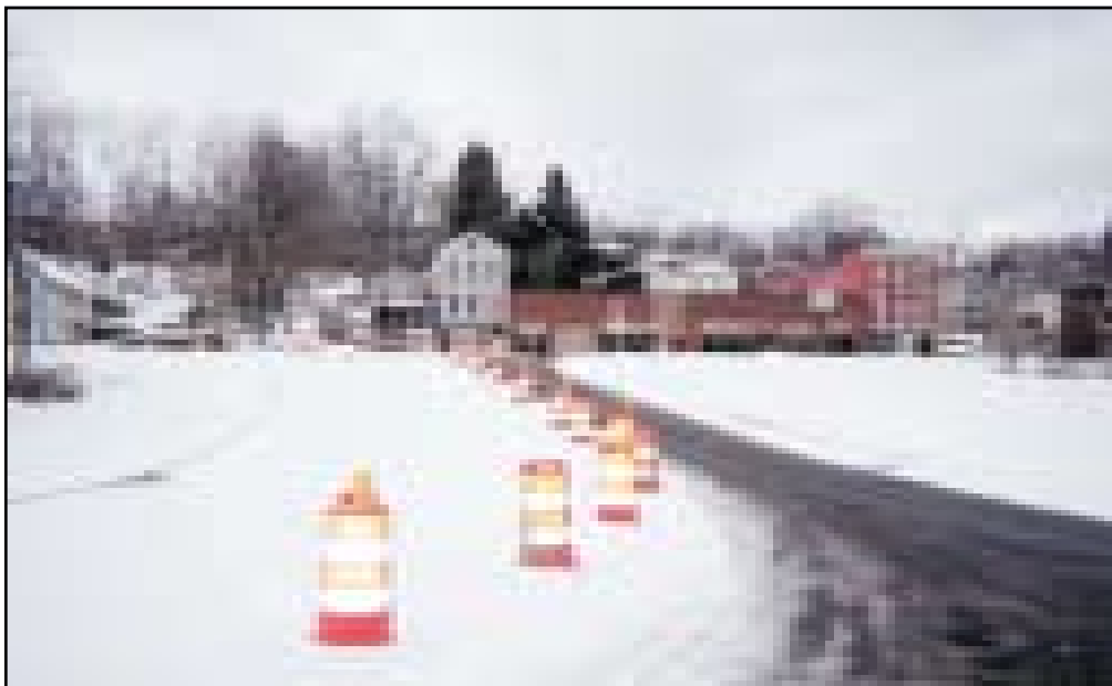
This photo shows the "Farley Connector", a stretch of roadway that will connect the John B. Merrill Parkway (currently, River Street) with Main Street in Towanda. This connecting street was named in honor of the late Robert D. Farley, a long-termed Towanda Borough Councilman and President.
